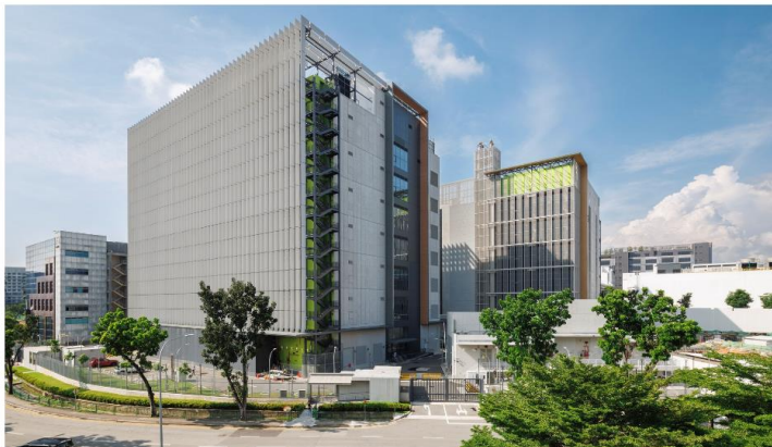
The two data centres, KDC SGP 7 and KDC SGP 8, are part of the Keppel Data Centre Campus at Genting Lane in Singapore.
